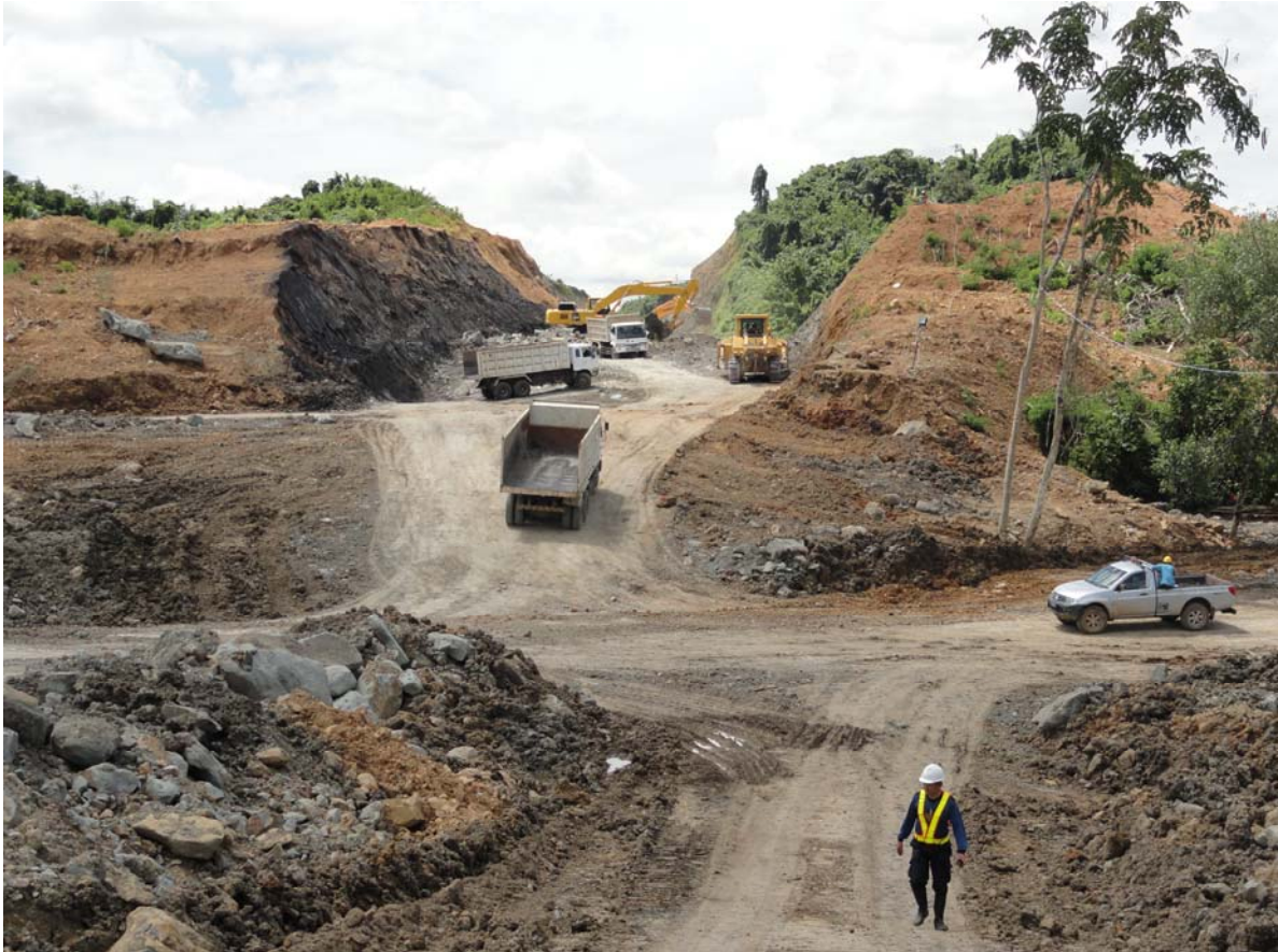
Overburden removal at Jongkang Mine.
